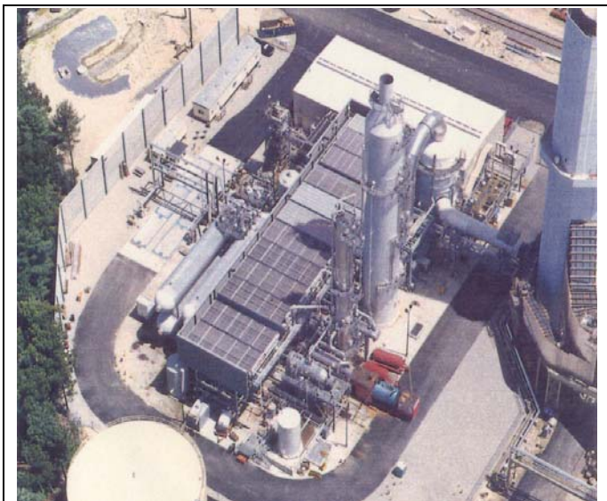
Proven CO 2 Recovery on Gas Turbine Exhaust; Bellingham Plant, USA - Aerial View (350 t/d) (Fluor Daniel)
